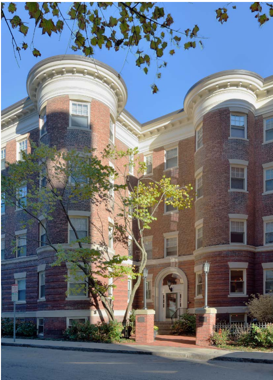
Photograph of Chapman Arms, taken by Joel Howe
