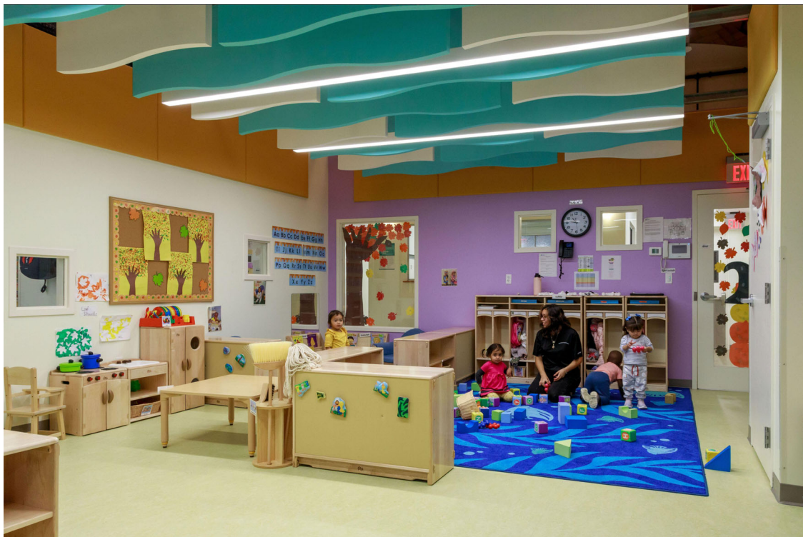
A classroom at the newly-renovated Barnes School operated by the East Boston Social Centers has wave-shaped acoustic tiles in the toddler classroom to help to buffer sound and diffuse light throughout the space. Poor acoustics in classrooms (due to high ceilings) can make it difficult for young children to hear each other and their educators, at a time when their language skills are rapidly developing. (Photo: Lynne Damianos)
